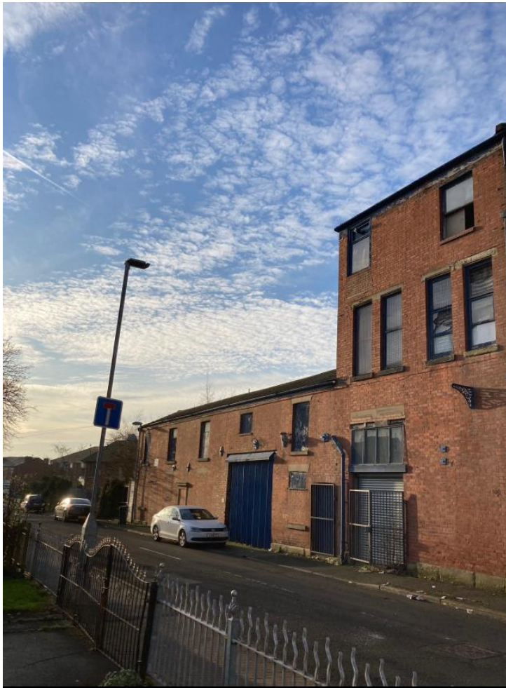
Photo 4: View of part of rear of building viewed from Bollington Street
